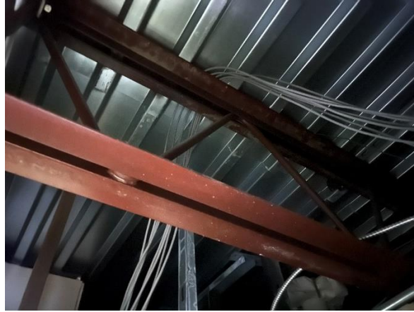
Photo 3: Underside of the roof deck in the general area of the stained ceiling tile in Photo 2 (above).
