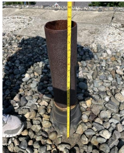
Photo 14: Roof flashing heights at the base of vent pipe.
