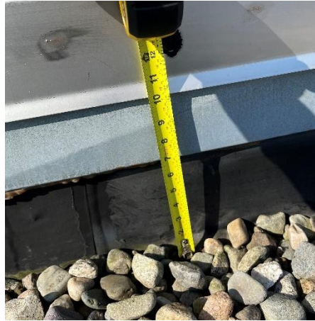
Photo 12: Rooftop equipment curb roof flashing height about 8 in. above the roofing membrane.
