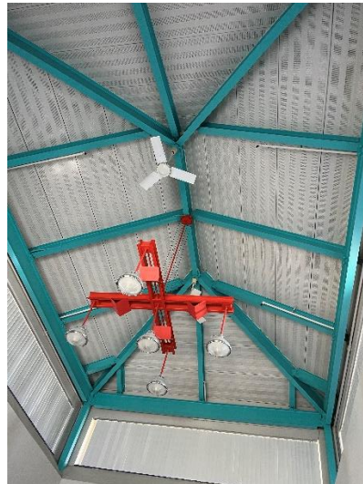
Photo 5: Overview of underside of hipped roof.
