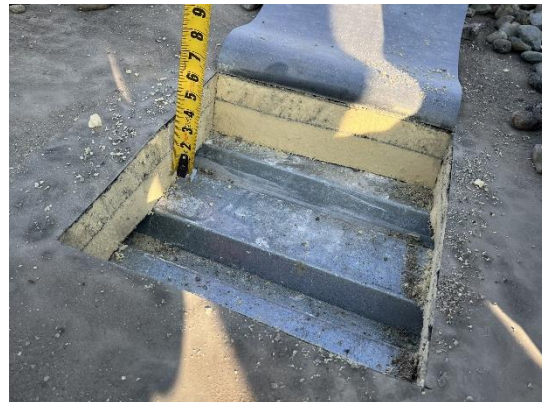
Photo 21: Typical Roofing system.
