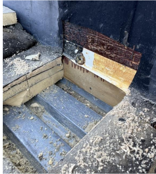
Photo 22: Roofing system at the base of a rising wall.
