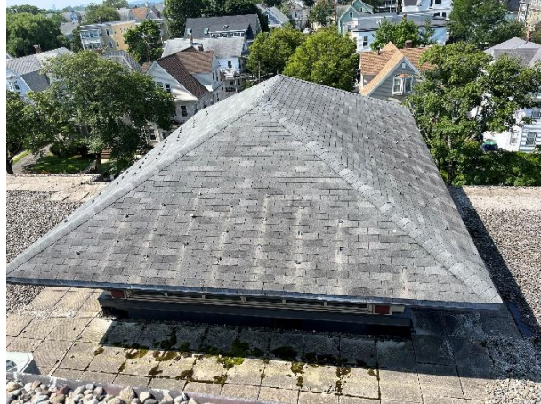
Photo 23: Overview of hipped roof covered with asphalt shingle roofing.
